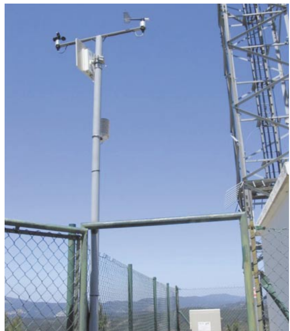
RADWIN's WinLink™ 1000 used for remote video surveillance of Portugal forest area
